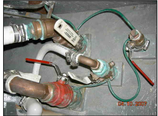
New sea valves, bonded
